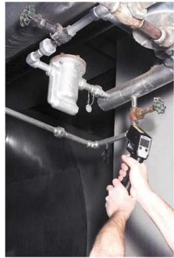
Steam valves are opened slowly to equalize pressure and warm the equipment downstream. This also allows steam traps to drain condensate so dangerous water hammer can be avoided.
