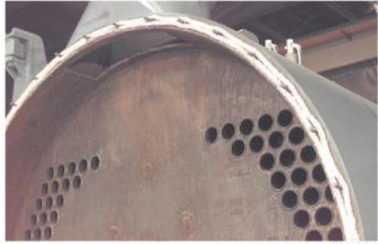
Frequently, the boiler inspector requires all of the plugs removed at the water column and the low water fuel cutoff controls opened so the inside float chamber can be inspected. Fusible plugs must be replaced. After both the fire side (means of heating the water) and water side of the boiler have been cleaned, notify the inspector that the boiler is ready for inspection.
