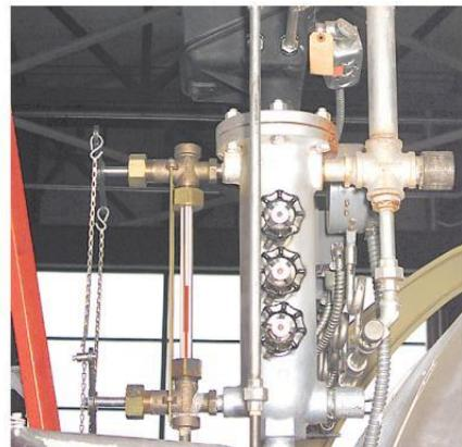
Ensuring the correct water level may be the most important duty of an operator. The gauge glass is the primary device used in determining water level and must be maintained and kept clean. It is connected to the water column which levels out the turbulent water in the boiler so it can be accurately read.
